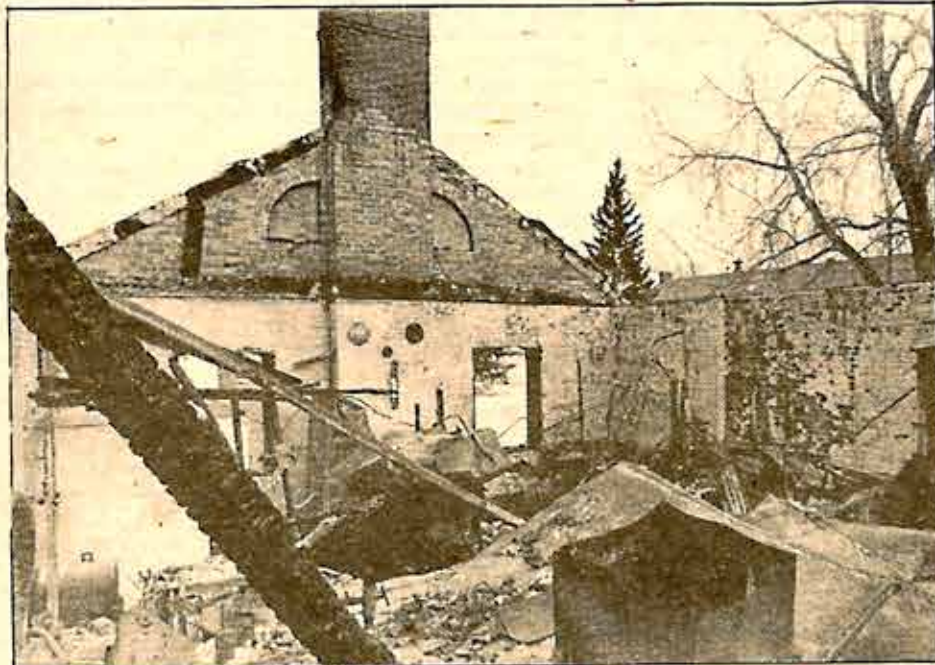
Only scorched brick walls remain after the blaze.
