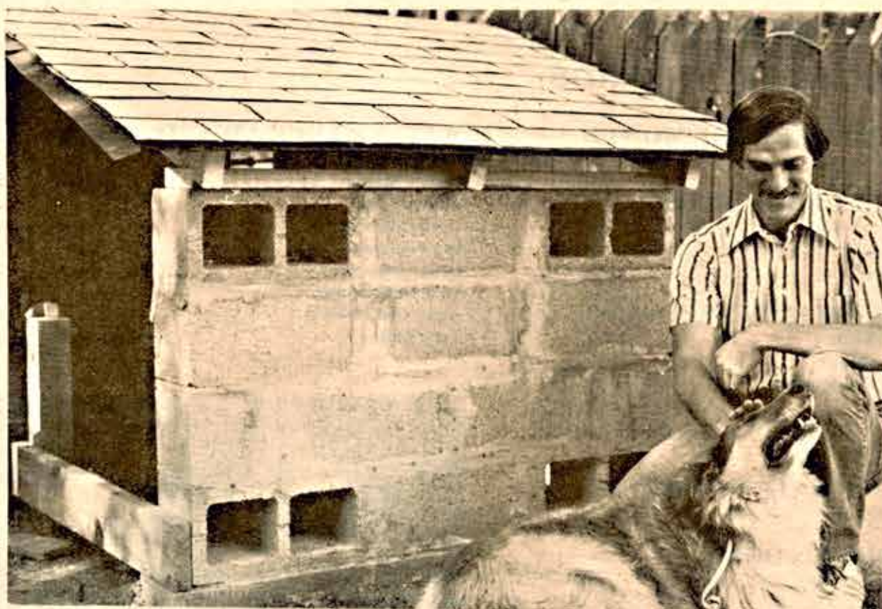
Arizona's first solar doghouse? - Andy Marshall thinks so, but it's also a pilot project in carefully measuring solar heating capabilities in the Ganado area. The cinder wall block, when painted black and covered with plastic, will absorb solar energy during the day and provide heat at night. Vents open and close allowing heat from the front to flow inside and keep the dog house and its occupant warm.
