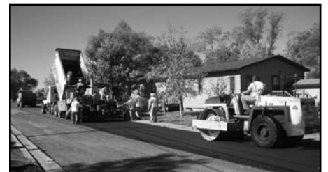
Paving Sisseton Street
