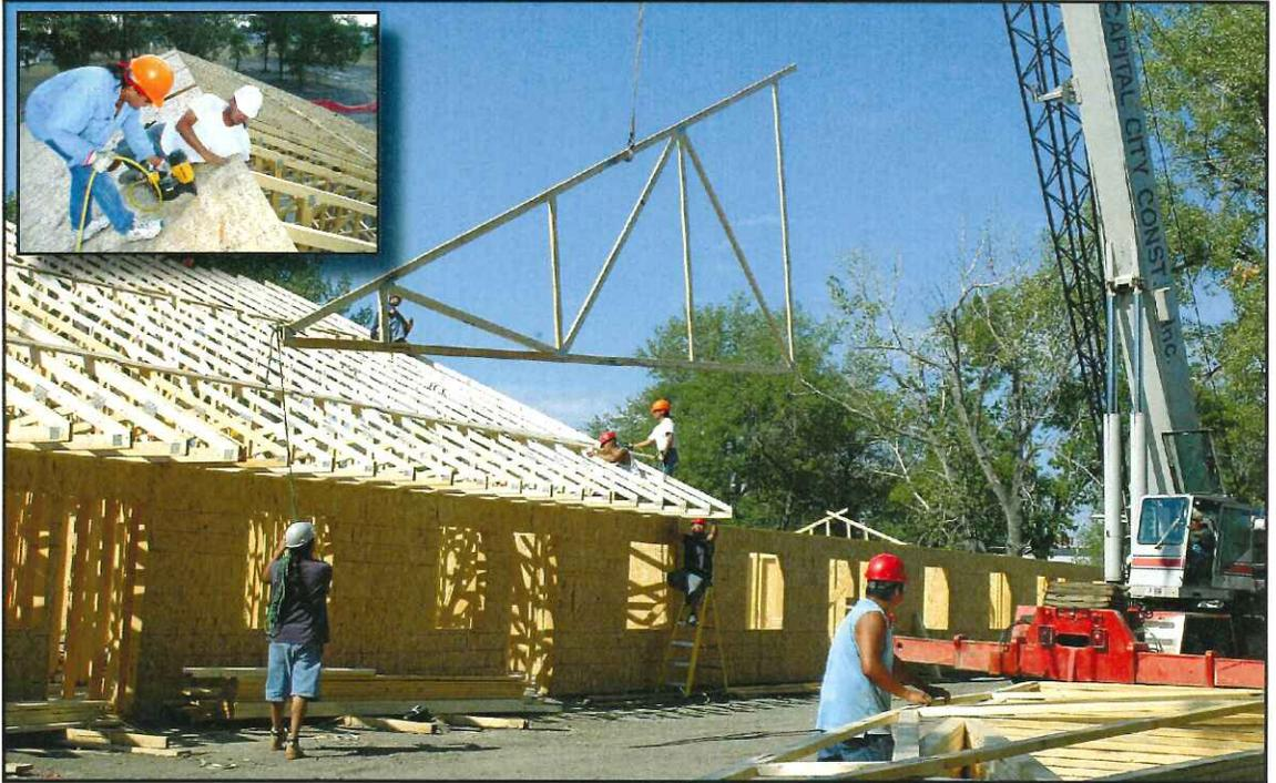
UTTC Construction Technology students assembled roof rafters for a new apartment complex during hot days in July when the temperature soared over 100 degrees. UTN photos Dennis J. Neumann
