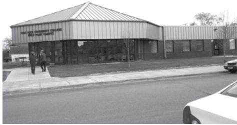
FPC campus at Wolf Point, MT
