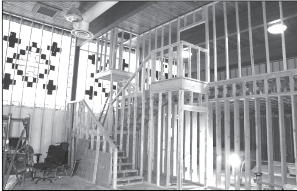
Space under construction for CCCC's HVAC training
