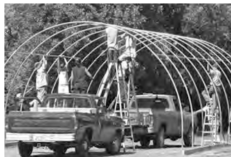
Hoop House raising, Dennis J. Neumann photo
