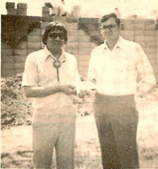
Francis Forster, president of Farmer's State Bank, Richardton, presents award to UTETC Executive Director Dave Gipp which will enable UTETC to purchase support equipment for the new Community Service Building. (Background shows construction now underway)
