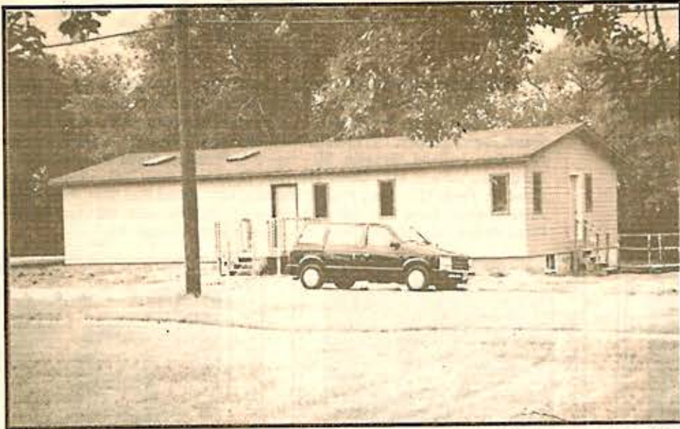
The New Cultural Arts and Gallery Building is near completion, except for the finishing touches. It is phase one of the United Tribes Arts Programs and houses the initial gallery, along with classrooms for the Art Entrepreneurial degree program, as well as the United Tribes self-sufficiency Telemarketing program. The building was constructed by the Building Trades students under the direction of instructor Eugene Staudinger. (UTTC Photo)
