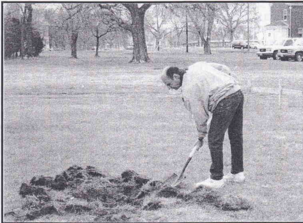
Wayne Pruse, Arts Faculty, was among those to break sod on the Great Plains, for a new Interpretive Arts Center on April 26, 2000. The log structure will be raised May 22, 2000 by volunteers.
